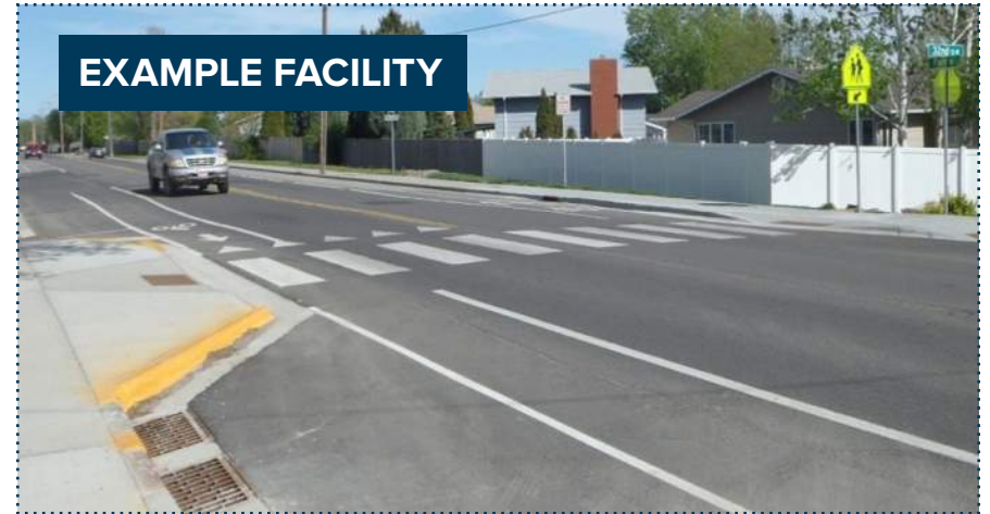
Example mid-block crossing with curb extensions and a striped crosswalk. Warning signage should be included ahead of the crossing in both directions, and an RRFB can be added if traffic volumes determine a need.
