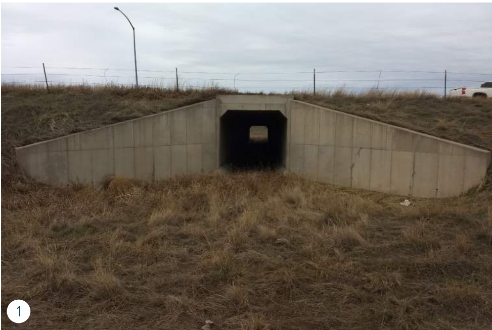
The existing cattle underpass should be considered for a trail underpass if it is determined to meet an acceptable standard. This underpass has less headroom than recommended.
