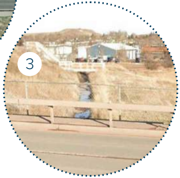
3 Difficult to cross drainage culvert
