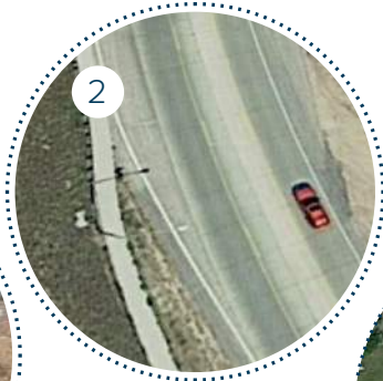
Wider sidepath needed to accommodate pedestrians and bicyclists
