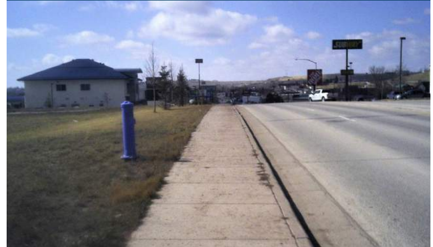
Sidewalk along Boxelder Road east of Cliff Davies Drive
