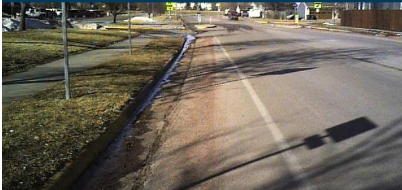
Paved shoulder on Harder Drive north of W Lakeway Road
