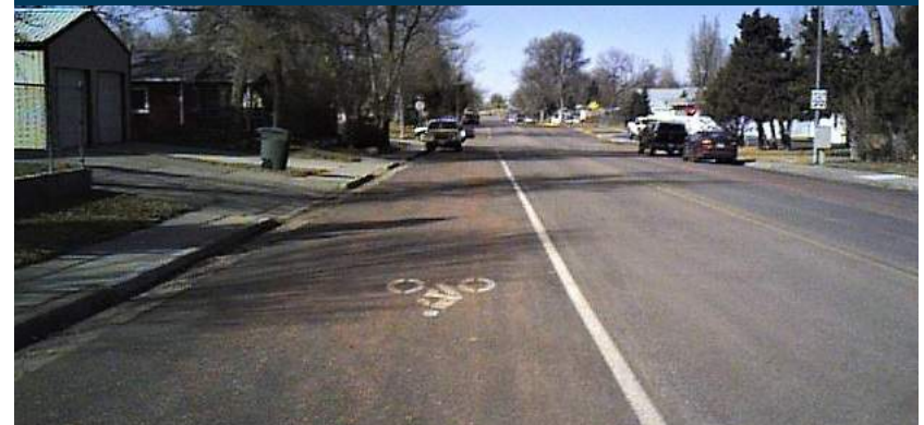
Bike Lane on S Brooks Avenue at E 8th Street
