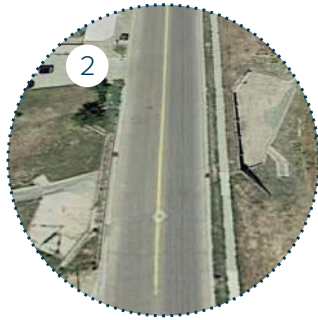
Mid-block crossing needed on Burma Ave.
