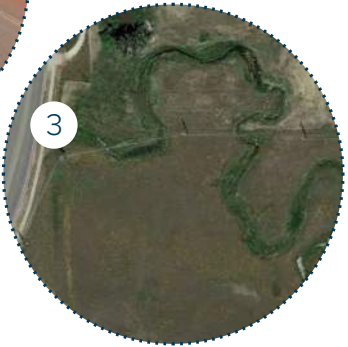
Pathway will need to cross drainage culvert
