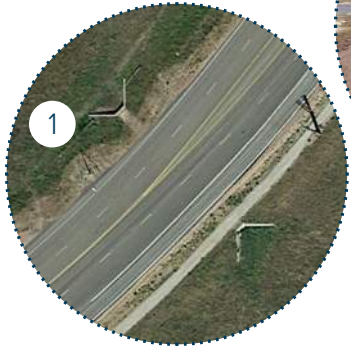
Existing cattle underpass could be used for a pathway underpass if feasible
