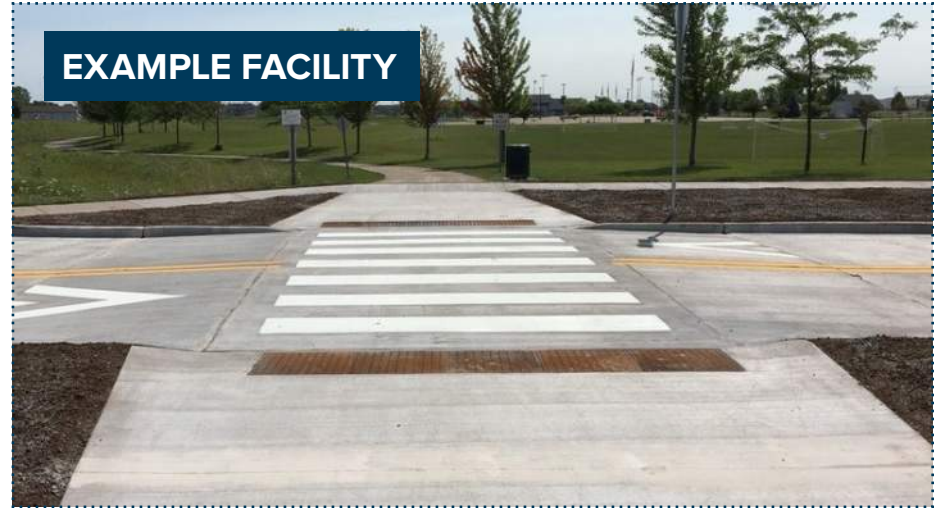
Example of a raised crossing which could be implemented at the entrance to the Gillette Golf Club to highlight the trail crossing
