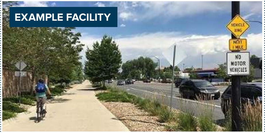
Sidepaths are wide pathways that run parallel to busy roadways. They provide a high-comfort, low-stress facility that is fully separated from vehicle traffic lanes.
