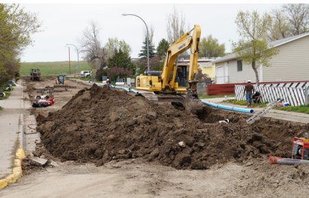
2015 Sanitary Sewer Main Replacement
