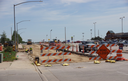
2018 Pavement Management Schedule B Camel Drive
