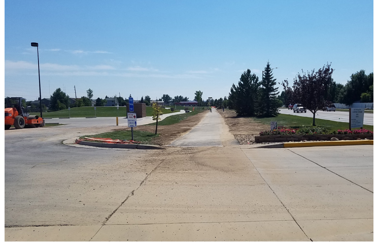
4-J Pathway Repair
