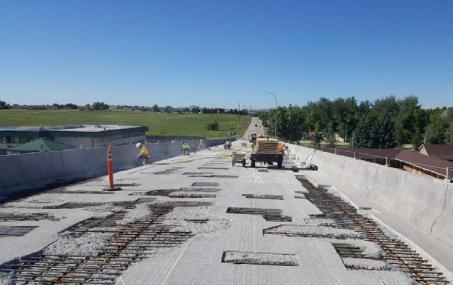
Gurley Overpass Deck Rehabilitation
