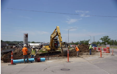
2018 Water Main Replacement
