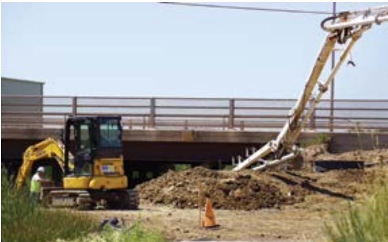
Dalbey - College Pathway Phase 1 (looking west)
