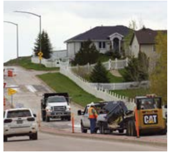
Large Patch Project (Force Road)
