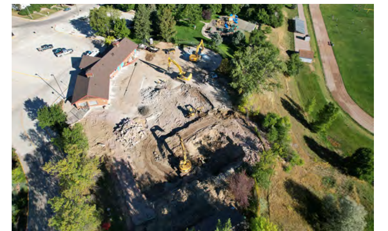
CITY PARK POOL DEMOLITION PROJECT $600,000
