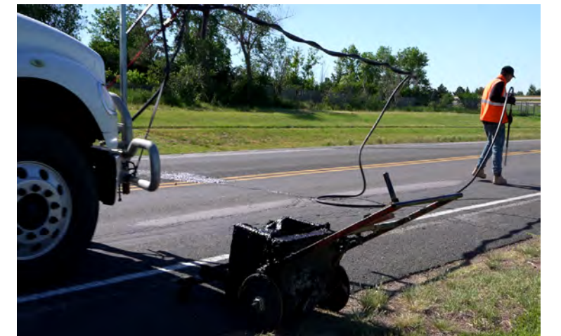
ANNUAL CHIP SEAL AND CRACK SEAL PROJECTS $450,000
