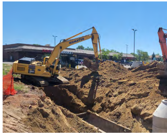
Fir Avenue Sanitary Sewer Repairs
