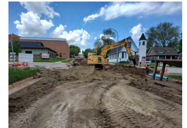
7th Street Water Main Replacement
