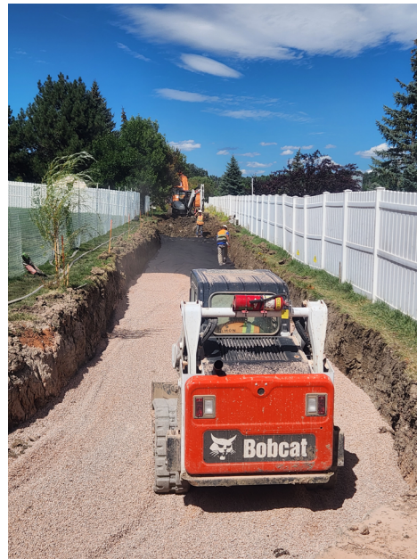
Lakeway Road Improvements
