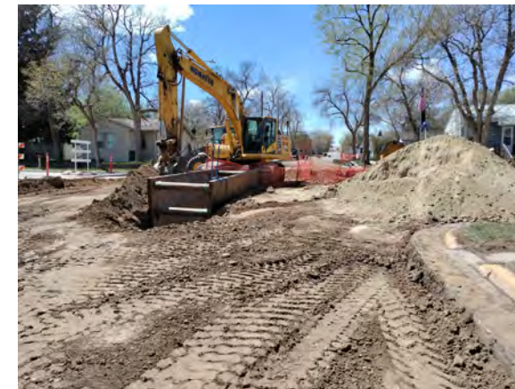
7th Street Water Main Replacement
