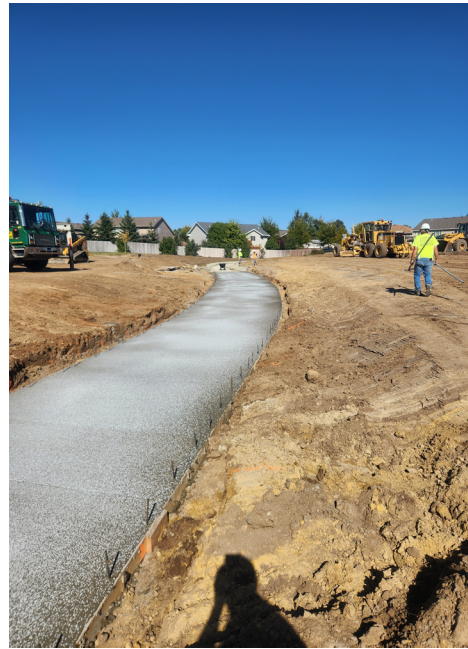
Providence Park Drainage
