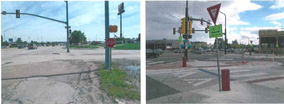
Left: Sidepath users along Douglas Highway have an unclear route across a busy intersection. Right: Right-turn bypass design in Boulder clarifies the pathway.
