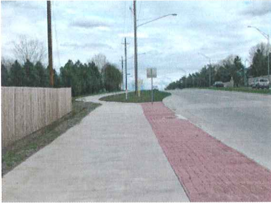
Sidepath along a major street uses contrasting paving where right-of-way is limited for visual separation, and moves away from the street when possible. Intersections are typically close to the intersection for maximum visibility.
