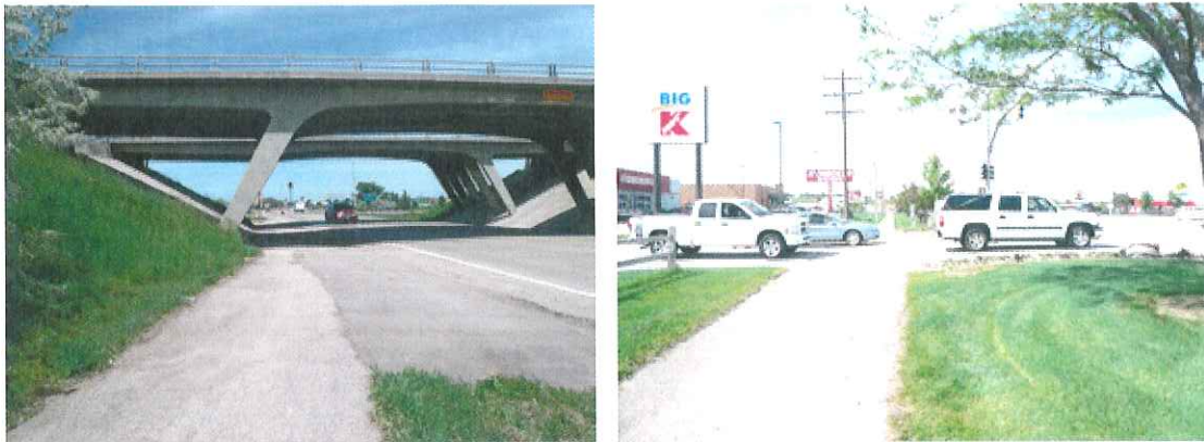
Sidepath Issues. Left: Sidepath under Interstate 90 is not well delineated from the main road and encourages counter flow bicycle traffic without adequate separation from the street. Right: Sidepath along Douglas Highway crosses streets and driveways well behind the roadway edge, obstructing visibility of path users and motor vehicles.
