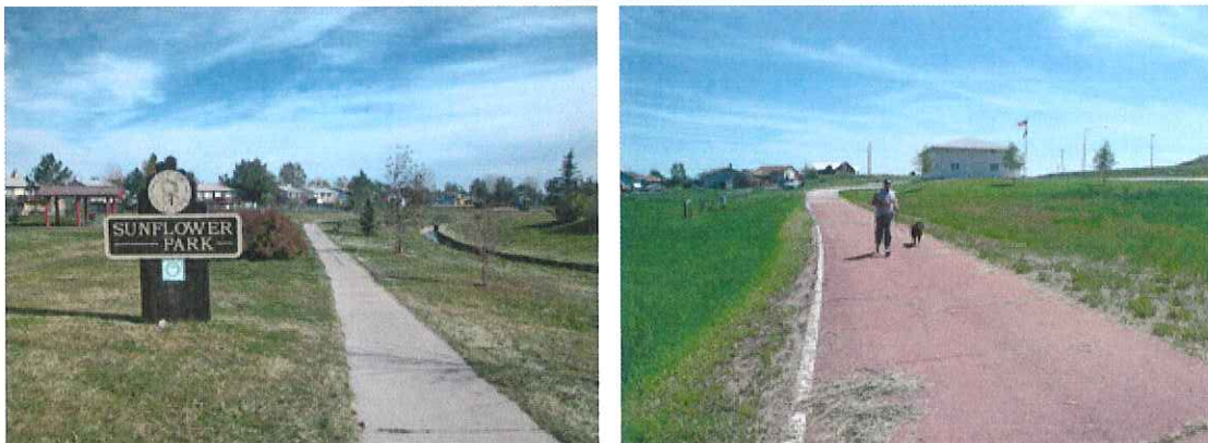
Multi-Use Trails. Left: Sunflower Trail connects the 4-J Trail with Sunflower Park and can provide access to major retail centers along Douglas Highway. However, the trail is too narrow to meet multi-use standards. Right: Trail paralleling West 4-J Road serves Sutherland Park but requires resurfacing and reconstruction in some areas.
